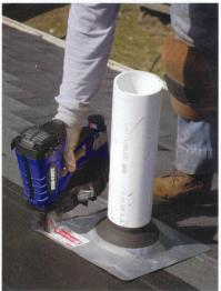
have to worry about dragging hoses through the wet tar, which makes a mess of the roof and the hoses." They have three of the nailers on the job and have been very successful in this application. The crews also use it on commercial jobs where they have to nail off gravel stop and metal edging, and they like the results.
